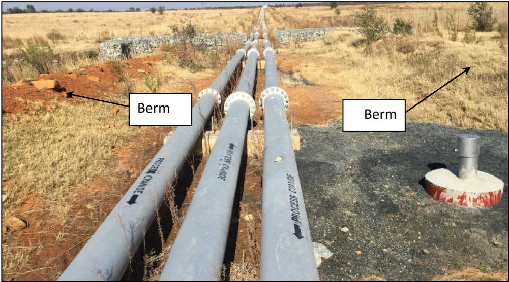
Figure 5: Spillage Trench
