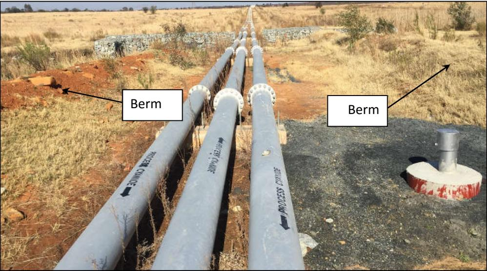
Figure 5: Spillage Trench
