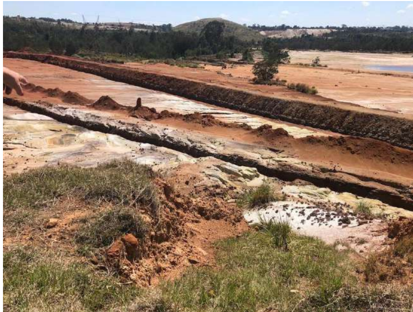
Acid mine water enters the Wonderfonteinspruit through unlined and unreclaimed pollution control dams on Mintails property. A Parliamentary investigation found a R460-million shortfall in the money needed for full cleanup. Photo supplied by FSE
