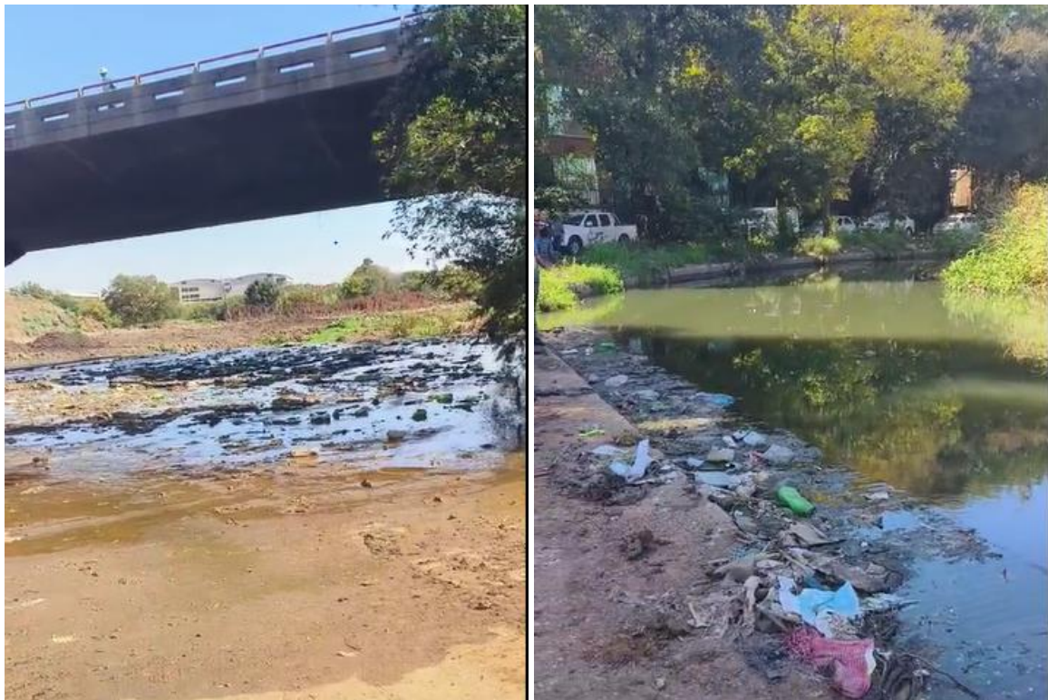
Significant raw sewage downstream of the Centurion Lake (Photo: Melissa Cronje)
